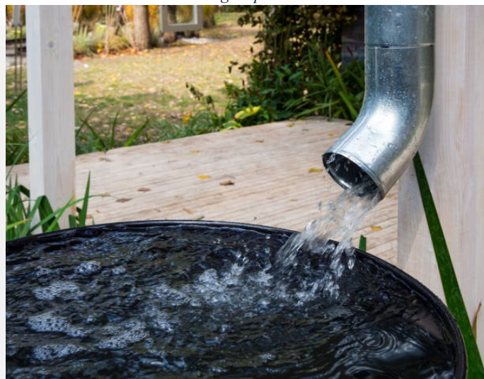
Figure 4. Rainwater or snow melt harvested in collection barrels can be used to irrigate plants and lawns
