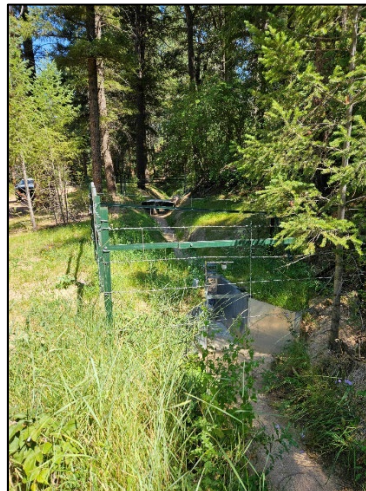
(New infrastructure along the Gove Creek irrigation ditch that measures and diverts water)
